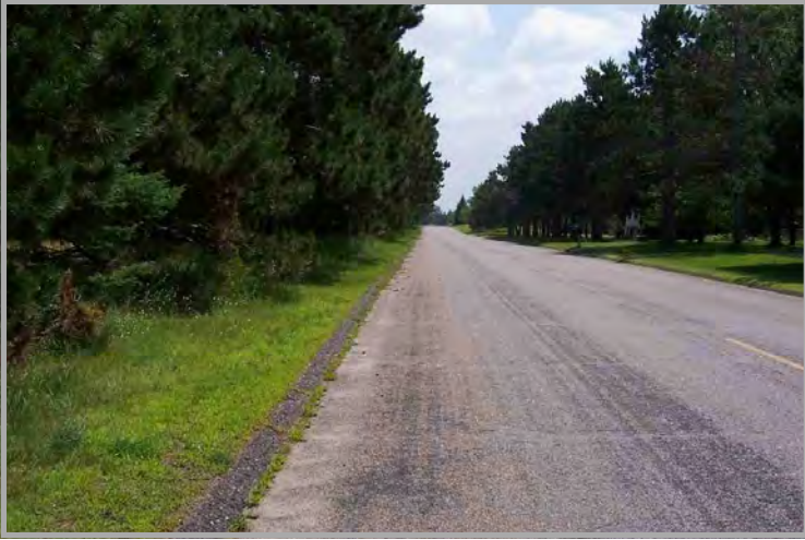
Street View Looking East
