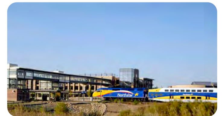
Northstar pulling into the Ramsey station
