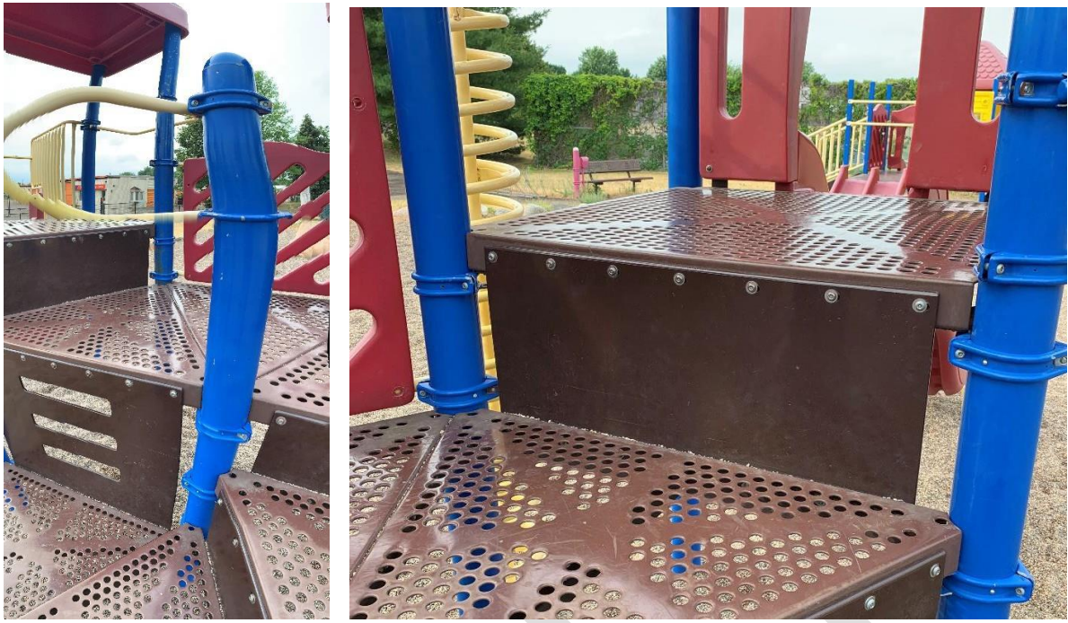
Figures 51-52: Transfer Surfaces on the Larger Playground at Riverdale Park (note that the picture on the left is a vertical panorama and is compressed vertically and angularly distorted)
