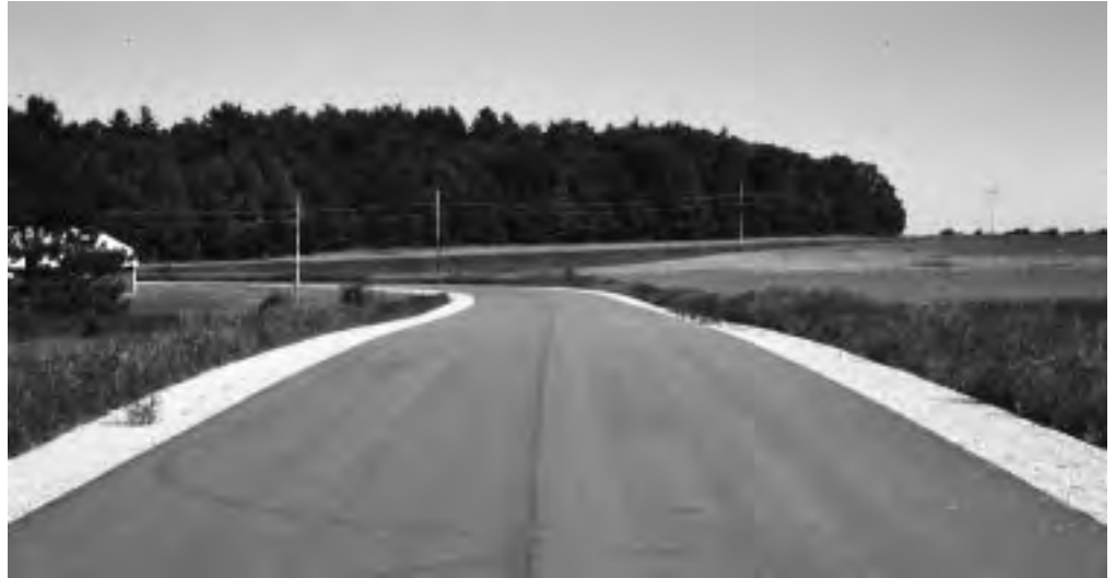
▶ RATING 10 New construction.
