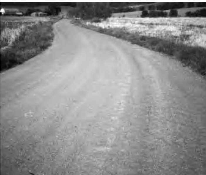
▲ New cold mix surface.
