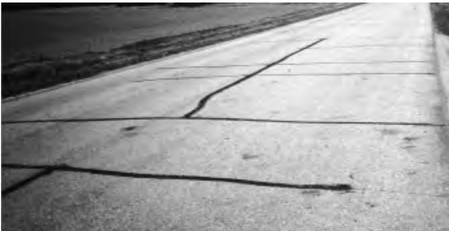
▼ Open crack, 1/2" wide; adjoining pavement sound.
