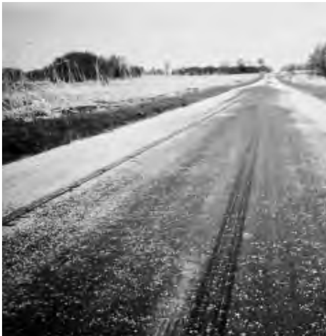
▼ Severe flushing.
