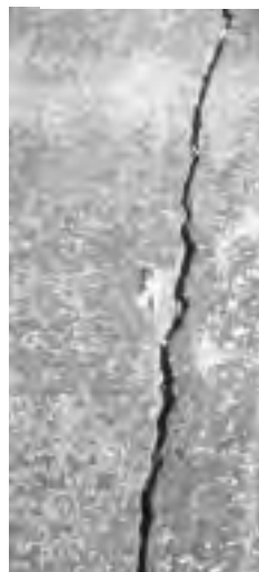
▼ Open crack, 1/2" wide; adjoining pavement sound.
