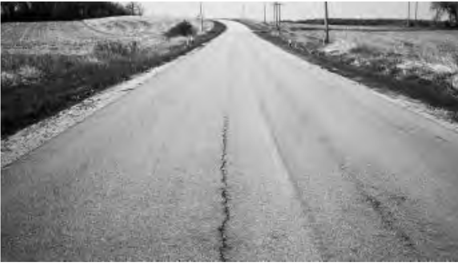
▼ Slight rutting; patch in good condition.
