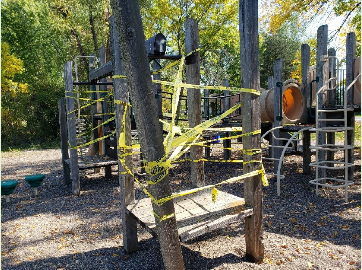
Peltzer Park – decayed posts (before September 2021 removal)
