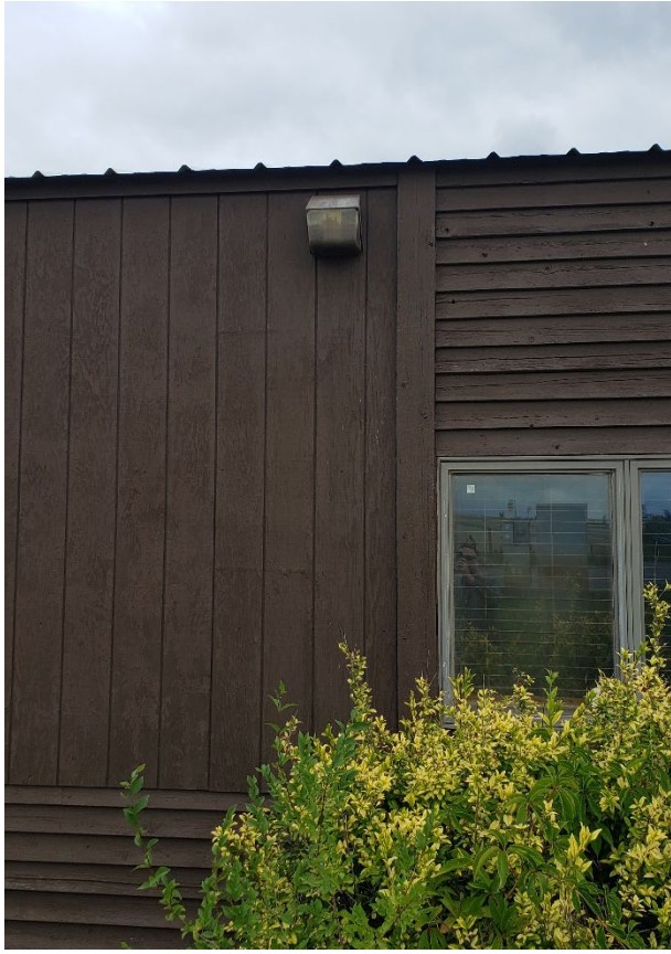
Photos 5 and 6. Existing wall-pack lighting proposed for upgrades (August 15, 2022).
