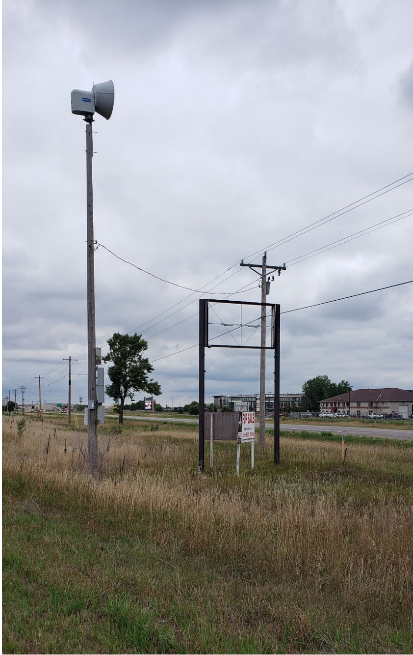
Photo 4. The proposed sign location looking westbound (08/15/2022).
