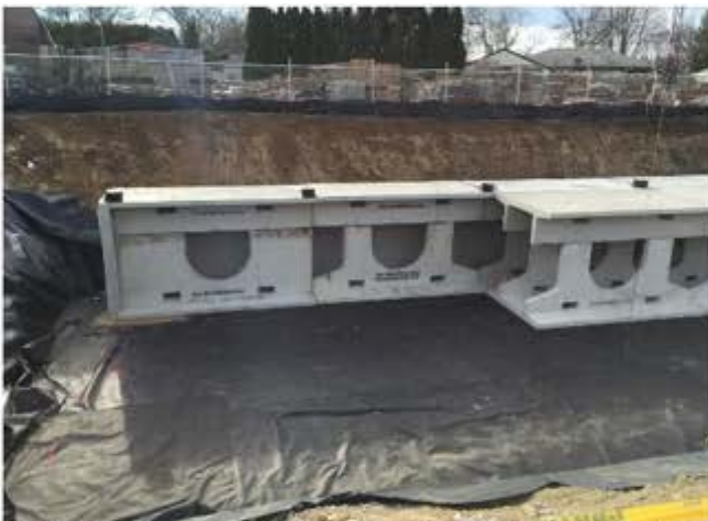
Exhibit 2: Example concrete vault storage tank (Storm Trap).
