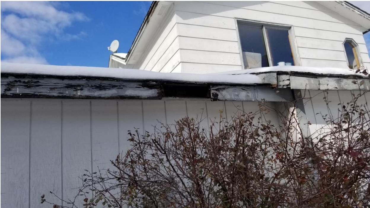
Photos Taken in October 2020 By Building Inspections Department
