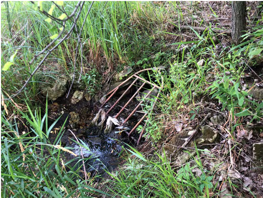
View of Wetland 2 culvert.
