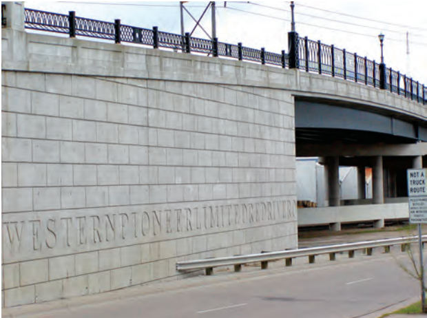
Selby Avenue bridge abutment. Michael Mercil.
