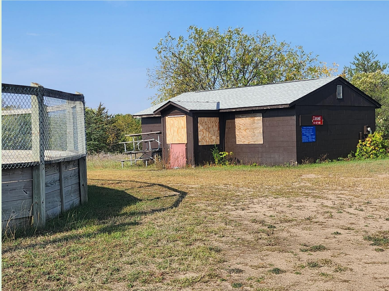
Ramsey Elementary School Warming House
