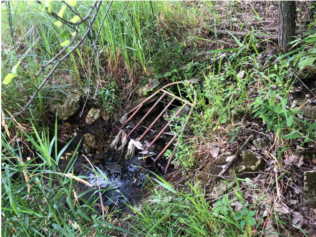
View of Wetland 2 culvert.
