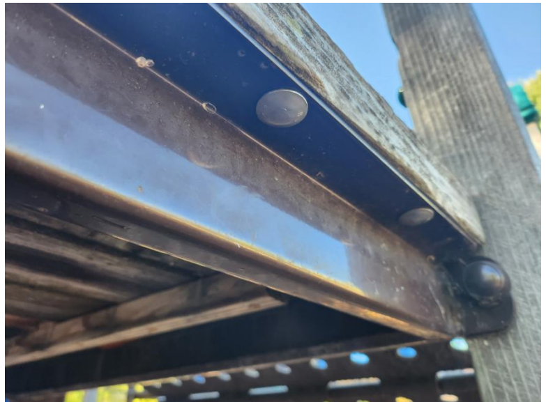
Bottom side of same deck fasteners
