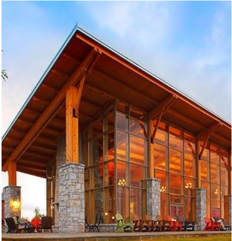
Heavy Timber Construction
