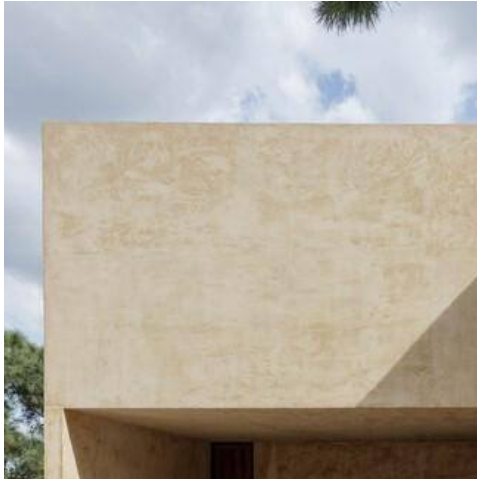
Exterior Plaster Finish
