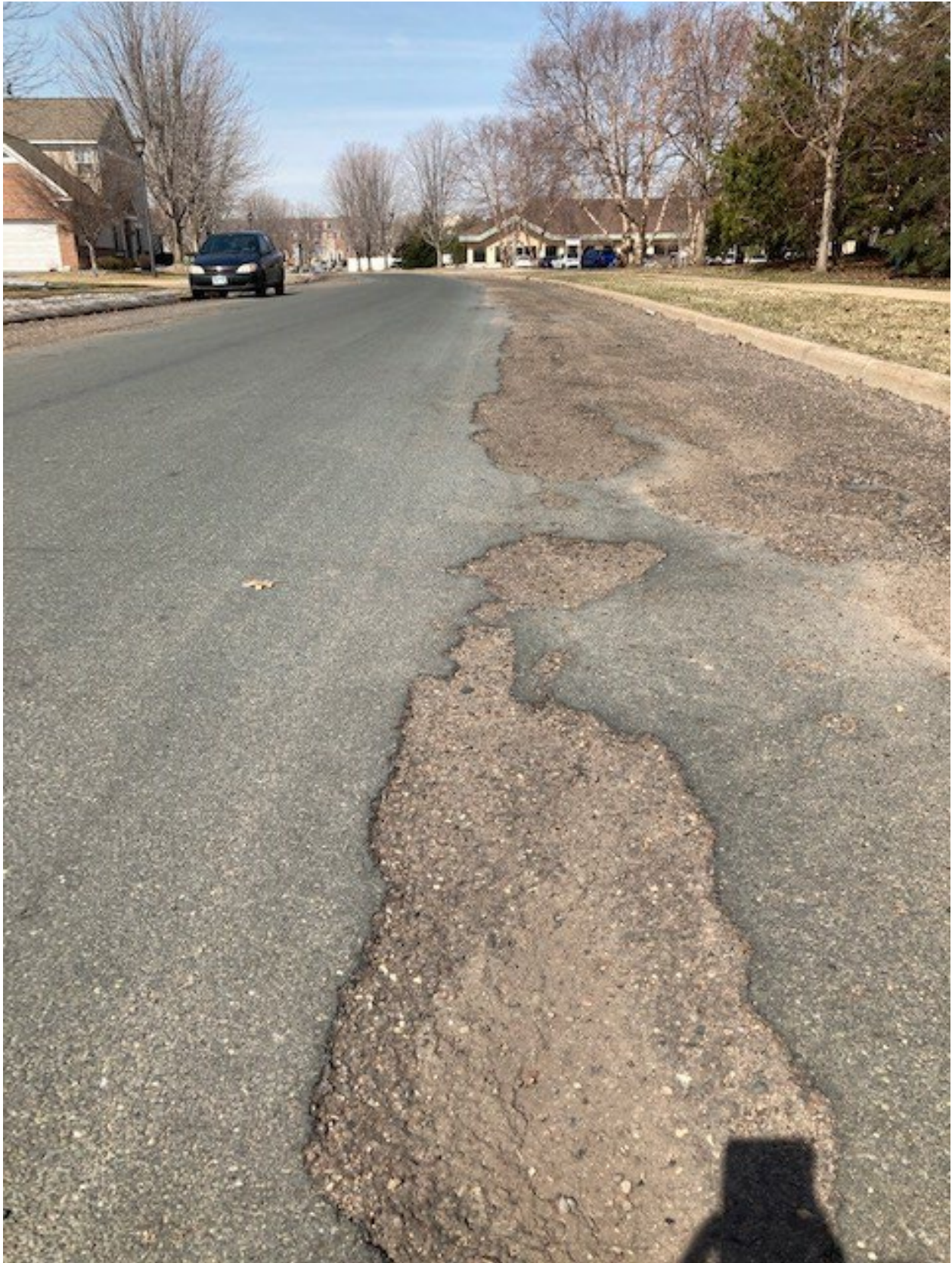
Figure 4 Rivenwick Village: Pavement Striping close-up
