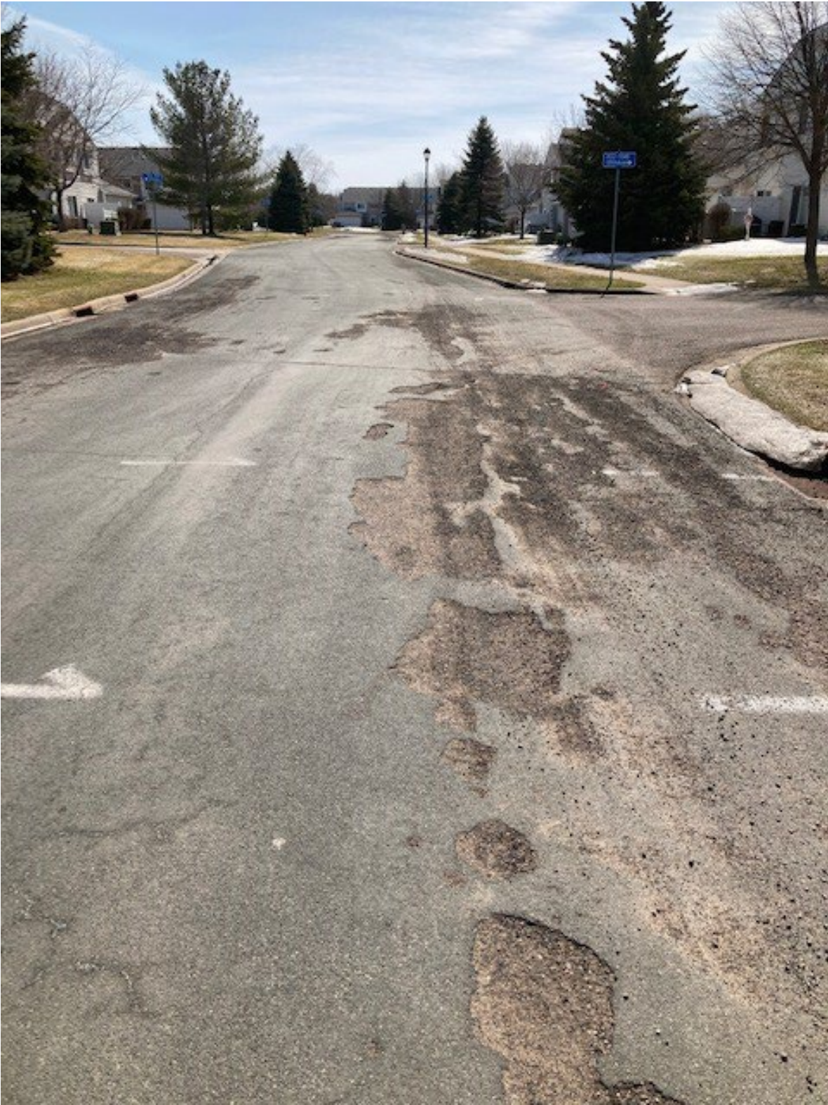
Figure 1 Rivenwick 3rd: 139th Avenue facing east
