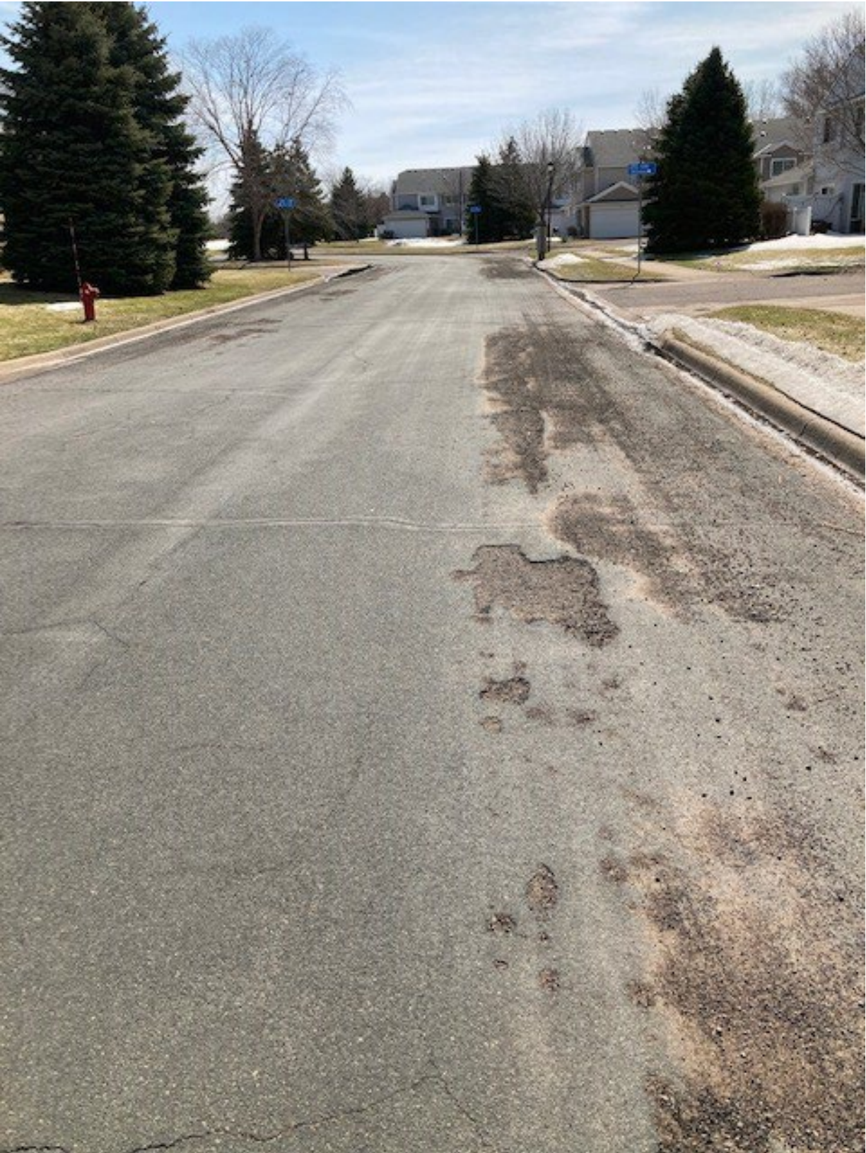
Figure 2 Rivenwick 3rd: 139th Avenue facing east
