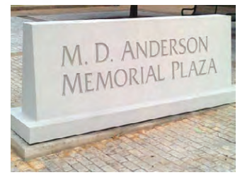
RECESSED LETTERING IN PRECAST CONCRETE
