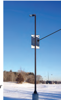
CITY STANDARD LIGHTPOLE SPACED 100' APART - ALTERNATING SIDES OF ROAD
