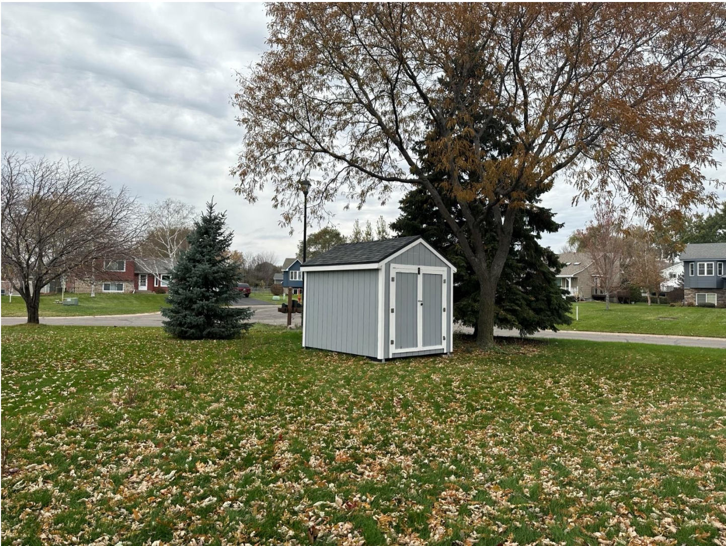
Picture of shed, looking northwest from the front of the house.
