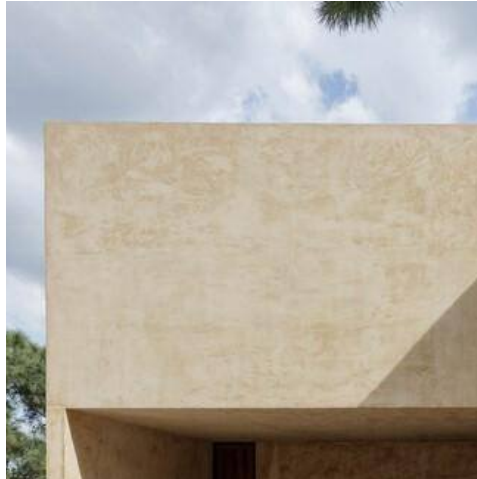
Exterior Plaster Finish
