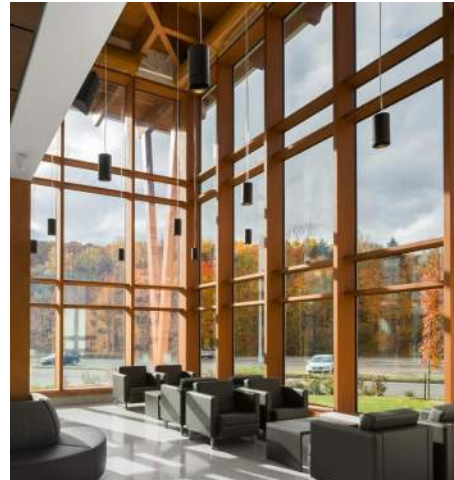
Timber Curtain Wall
