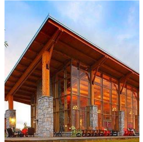
Heavy Timber Construction
