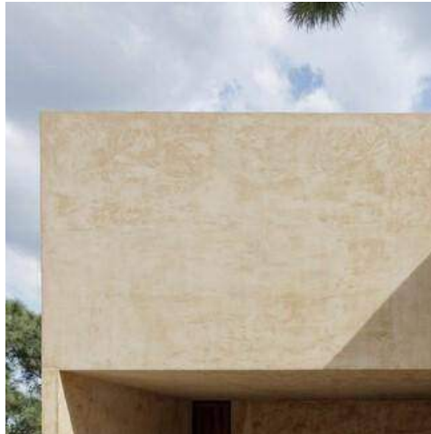
Exterior Plaster Finish
