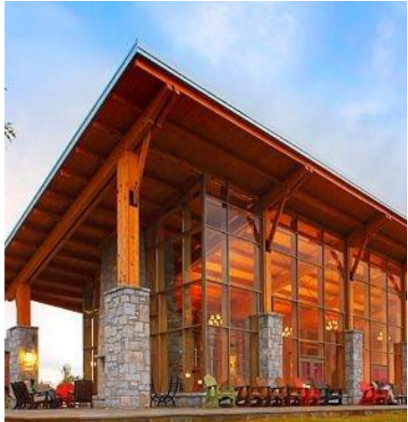
Heavy Timber Construction
