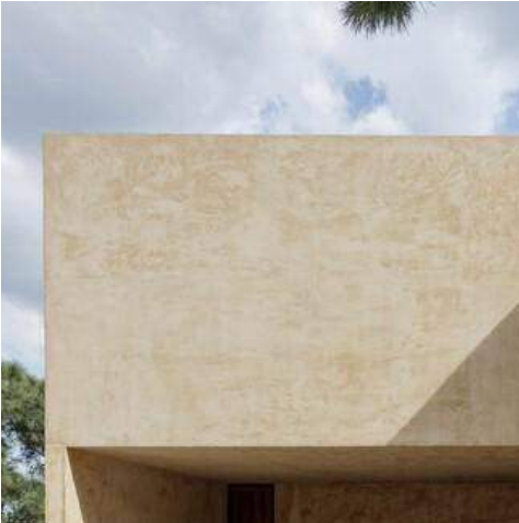
Exterior Plaster Finish
