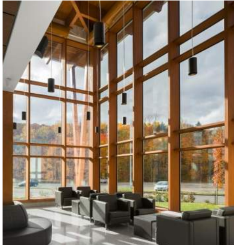
Timber Curtain Wall
