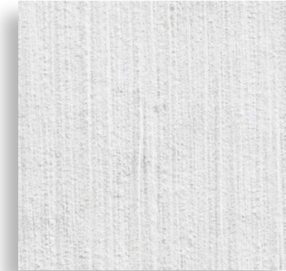
Light Broom Finished TILT-UP CONCRETE EXAMPLE
