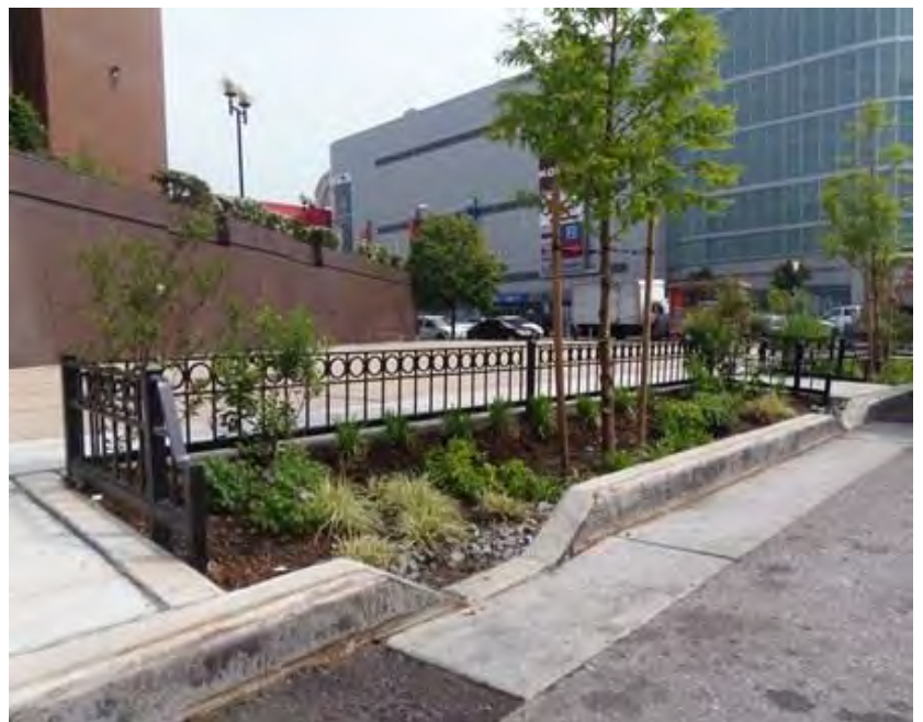
Figure 6: Right-of-way bioswale installed in New York City (NYC Environmental Protection, 2013)
