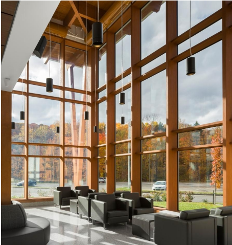
Timber Curtain Wall
