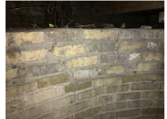
Figure 40 – Clay Masonry Wall
