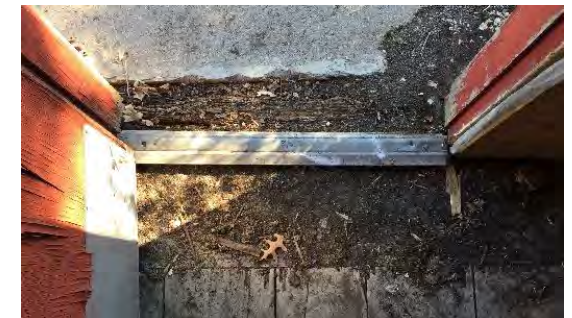
Figure 34 – Entry Hall Flooring at Threshold
