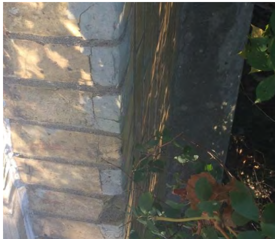
Figure 22 – Mortar Replacement to Fill Voids
