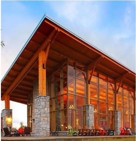
Heavy Timber Construction
