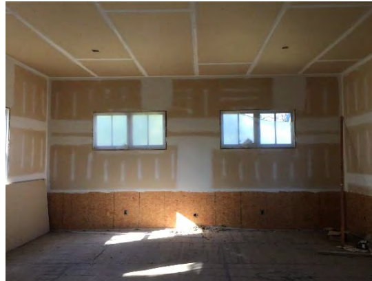
Figure 39 – Main Room, West Wall
