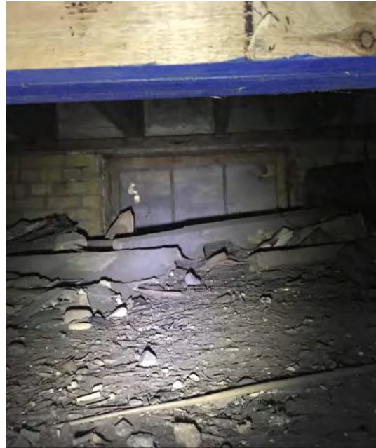
Figure 42 – Exterior Basement Window
