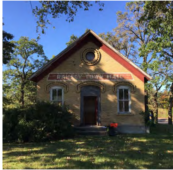
Figure 1 – Ramsey Town Hall Primary Façade
