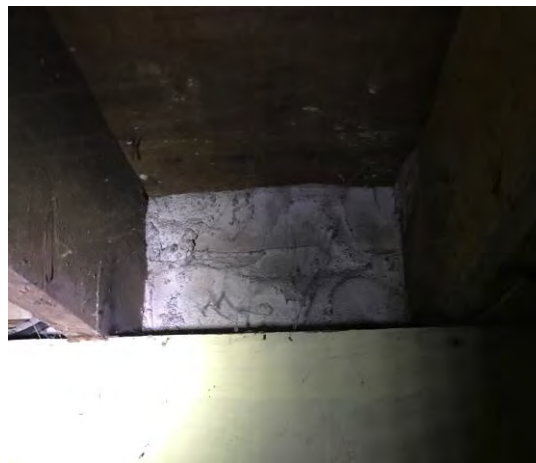
Figure 43 – Wall with Cementitious Material
