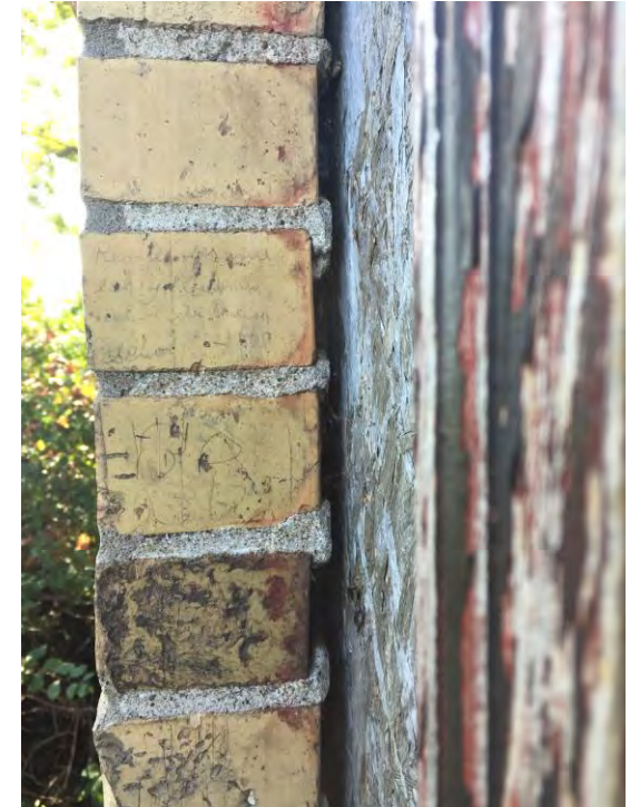
Figure 10 – Accessible Gap Behind Brick
