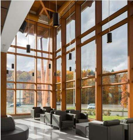
Timber Curtain Wall
