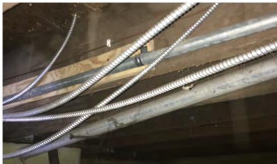
Figure 48 – Utilities Hole in Exterior Wall
