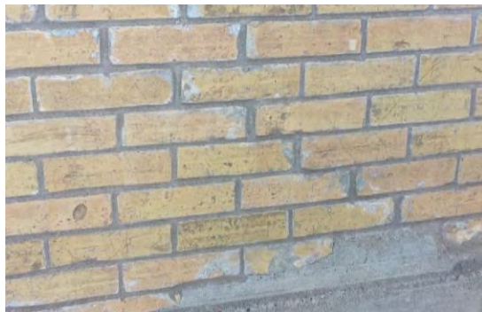
Figure 21 – Mortar Replacement to Fill Voids
