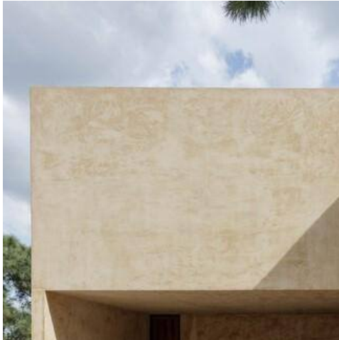
Exterior Plaster Finish
