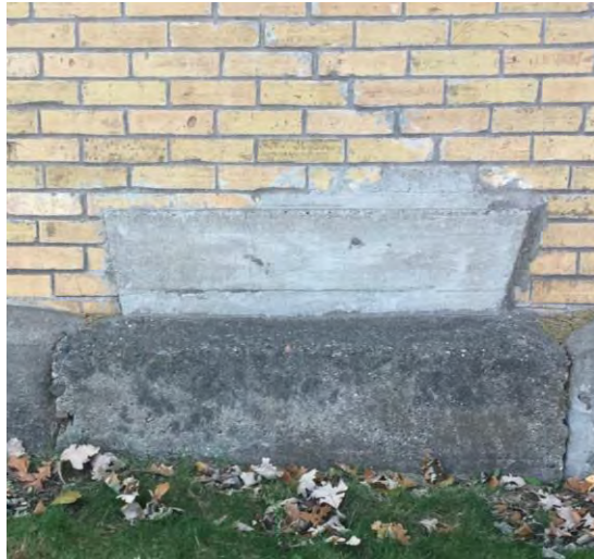
Figure 30 – South Elevation Window
