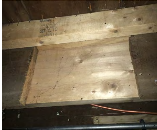
Figure 44 – Replacement Floor Joist
