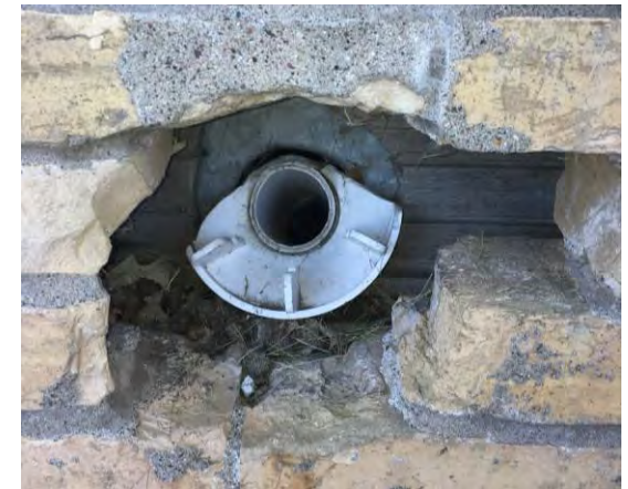
Figure 23 – Exterior Pipe Penetration
