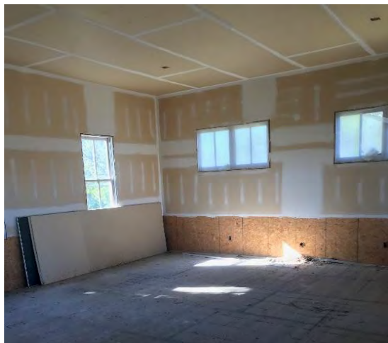
Figure 34 – Main Room, Northwest Corner
