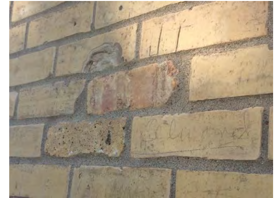
Figure 23 – Replacement Bricks
