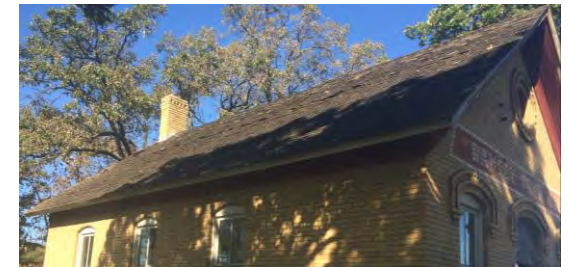
Figure 28 – Asphalt Shingles
