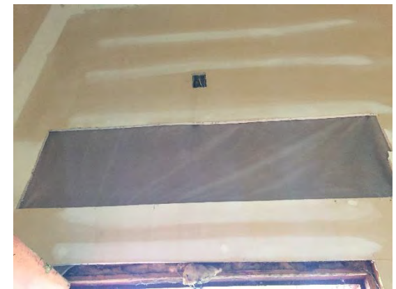
Figure 32 – Opening Above Entry
