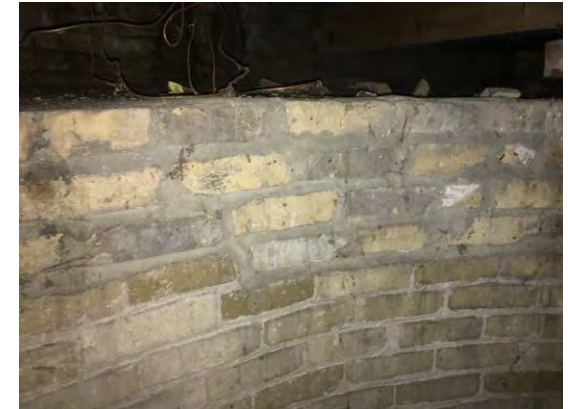
Figure 40 – Clay Masonry Wall
