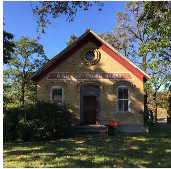
Figure 1 – Ramsey Town Hall Primary Façade
