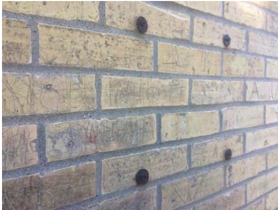
Figure 16 – Metal Brackets in Brick
