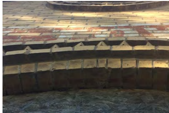
Figure 6 – Red Paint on Overhead Framing
