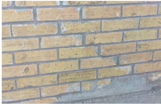
Figure 21 – Mortar Replacement to Fill Voids
