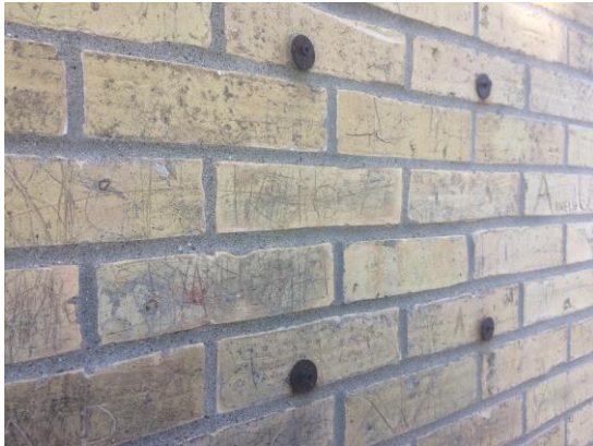
Figure 16 – Metal Brackets in Brick
