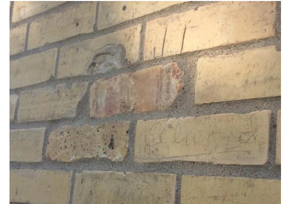
Figure 23 – Replacement Bricks
