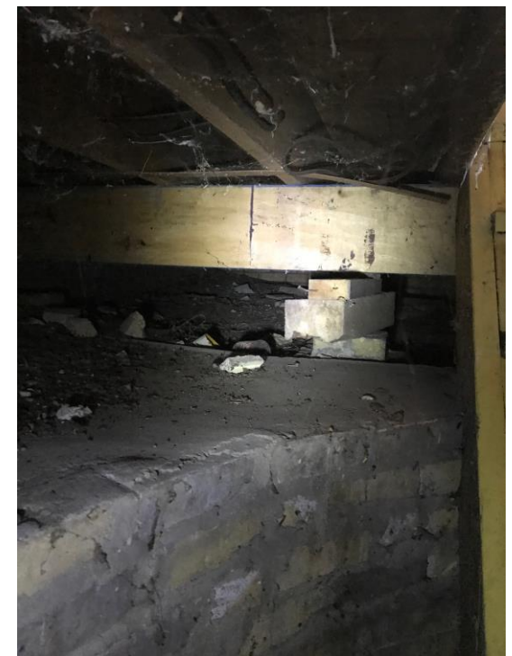
Figure 47 – Beam Support
