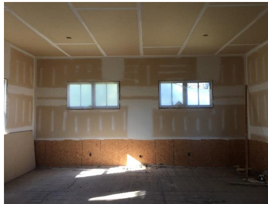
Figure 39 – Main Room, West Wall
