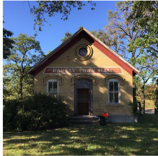
Figure 1 – Ramsey Town Hall Primary Façade
