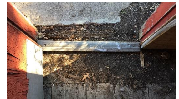
Figure 34 – Entry Hall Flooring at Threshold
