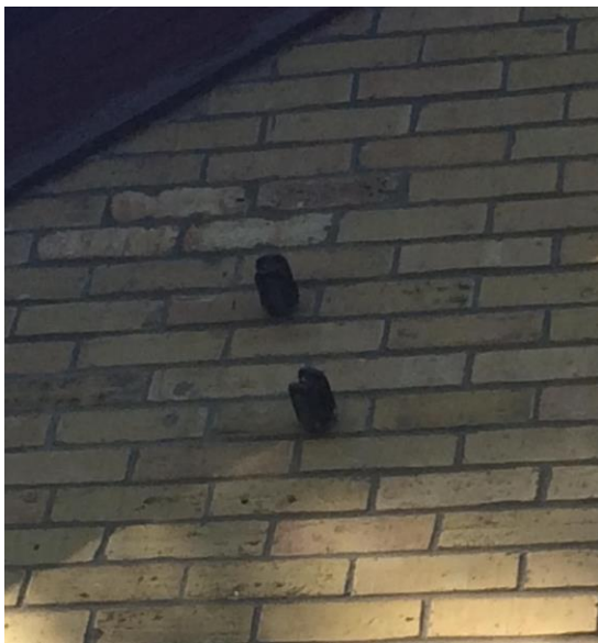
Figure 17 – Metal Brackets in Brick
