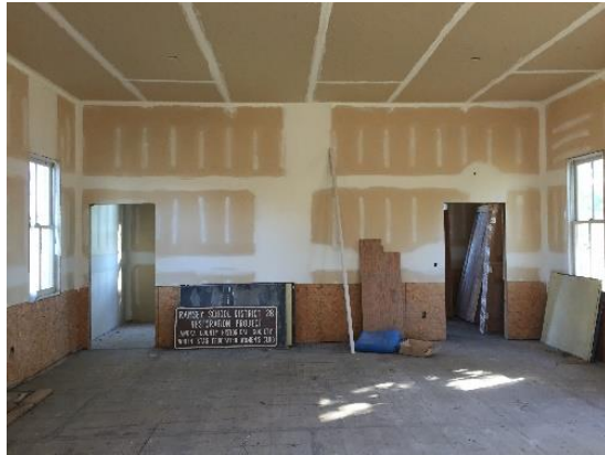
Figure 33 – Main Room, East Wall
