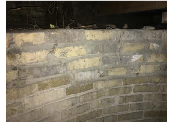
Figure 40 – Clay Masonry Wall
