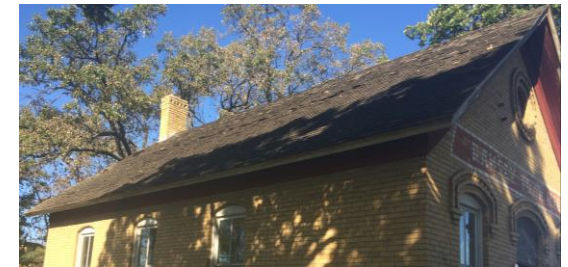
Figure 28 – Asphalt Shingles
