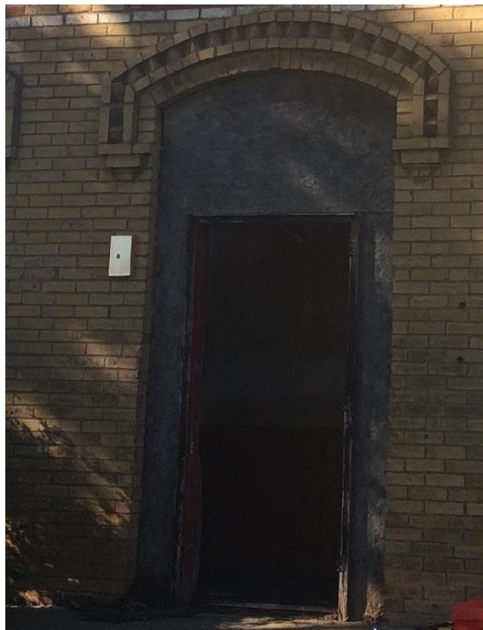
Figure 5 – Front Entrance with Particleboard
