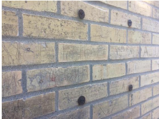
Figure 16 – Metal Brackets in Brick
