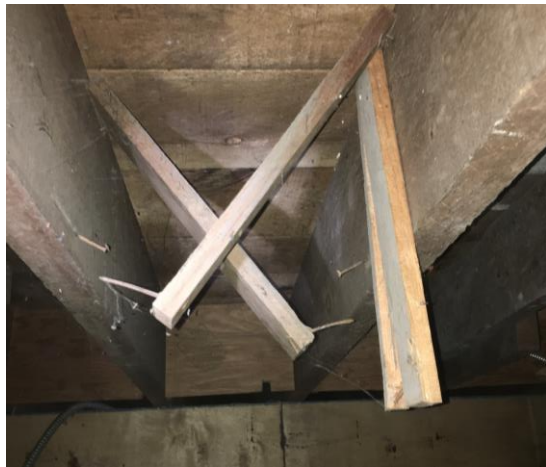
Figure 45 – Joist Cross Bracing
