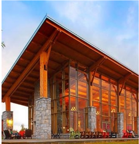
Heavy Timber Construction
