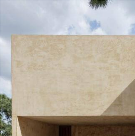
Exterior Plaster Finish
