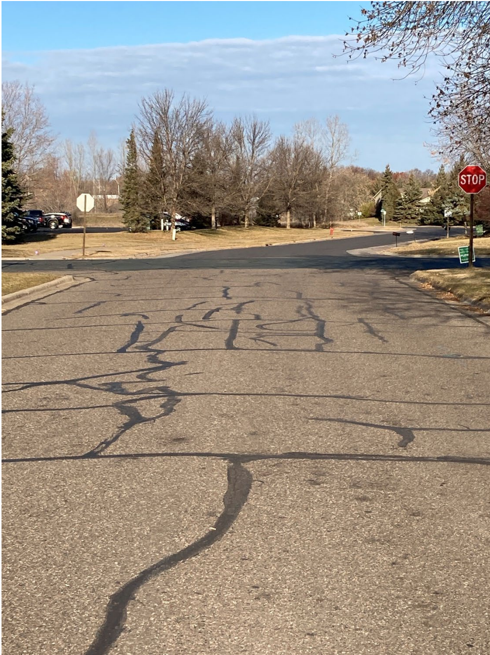
Xkimo Street: North of 142 nd Avenue, facing north
