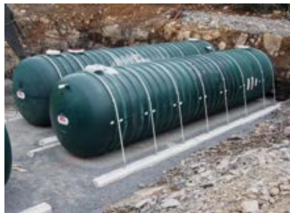
Exhibit 3: Example underground fiberglass storage tanks (Xerxes).
