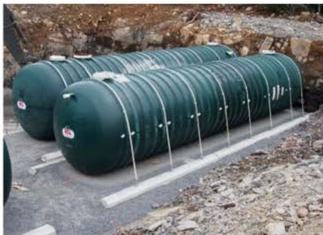
Exhibit 3: Example underground fiberglass storage tanks (Xerxes).
