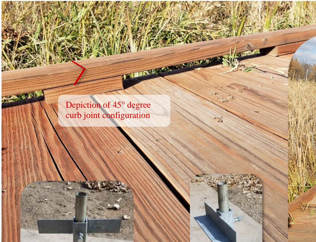
Example bracket hardware, mud foot plate and pipe
