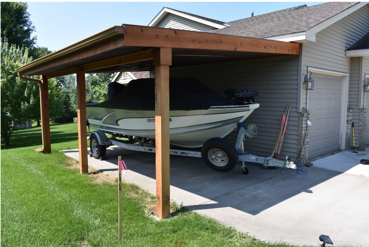
Photo 2. Looking southwesterly from the neighbor's yard.
