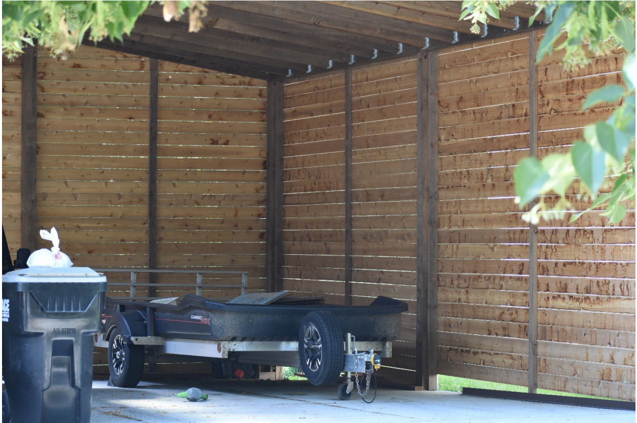
Photo 3. Views inside the structure from the applicant's driveway.
