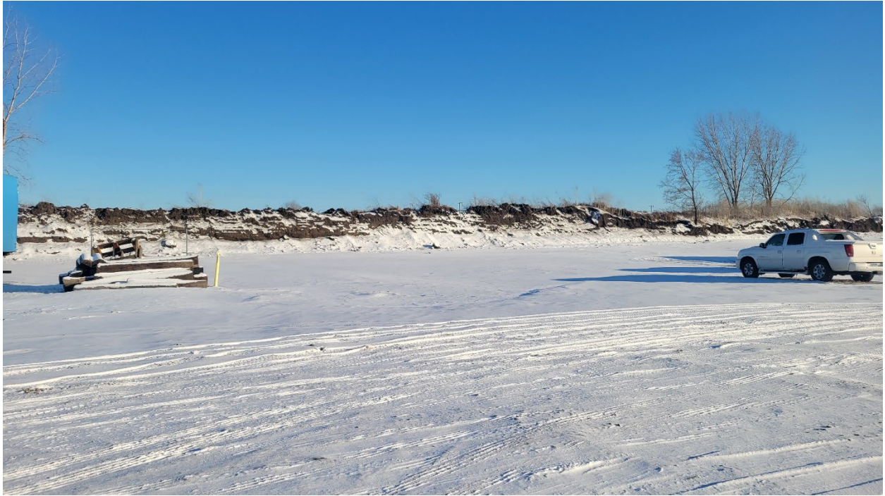
Photo 5. Looking southeast at the berm.
