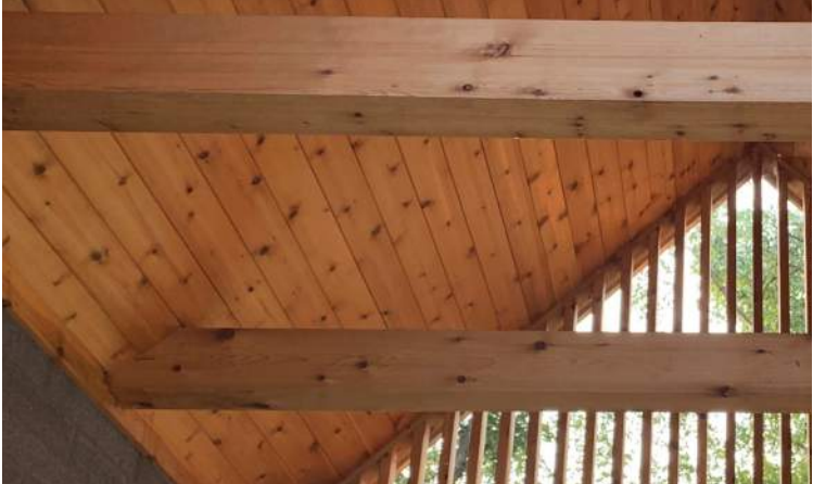
T&G Cedar Roof Underside Decking
