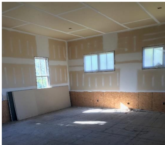
Figure 34 – Main Room, Northwest Corner
