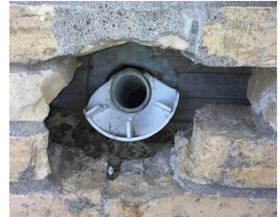
Figure 23 – Exterior Pipe Penetration
