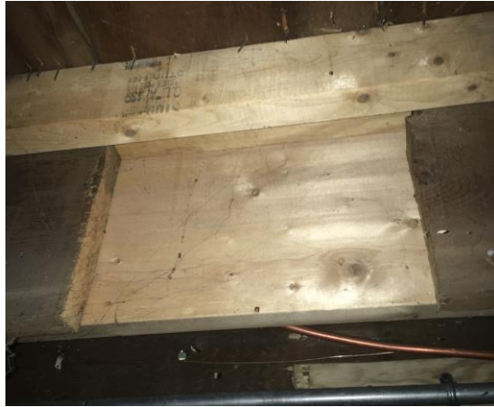
Figure 44 – Replacement Floor Joist
