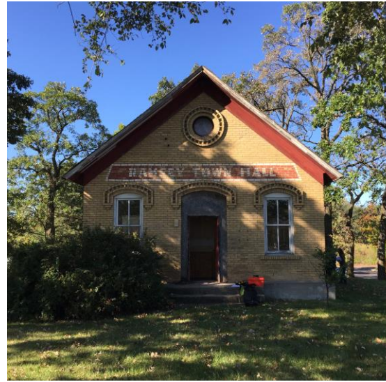
Figure 1 – Ramsey Town Hall Primary Façade
