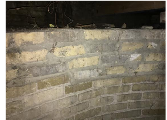
Figure 40 – Clay Masonry Wall
