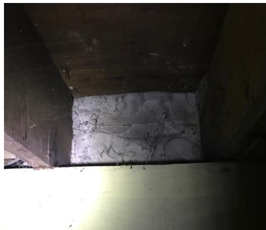
Figure 43 – Wall with Cementitious Material
