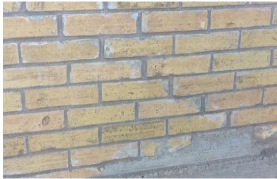
Figure 21 – Mortar Replacement to Fill Voids
