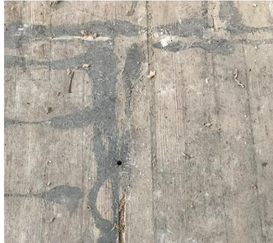
Figure 36 – Holes Along Wood Grain
