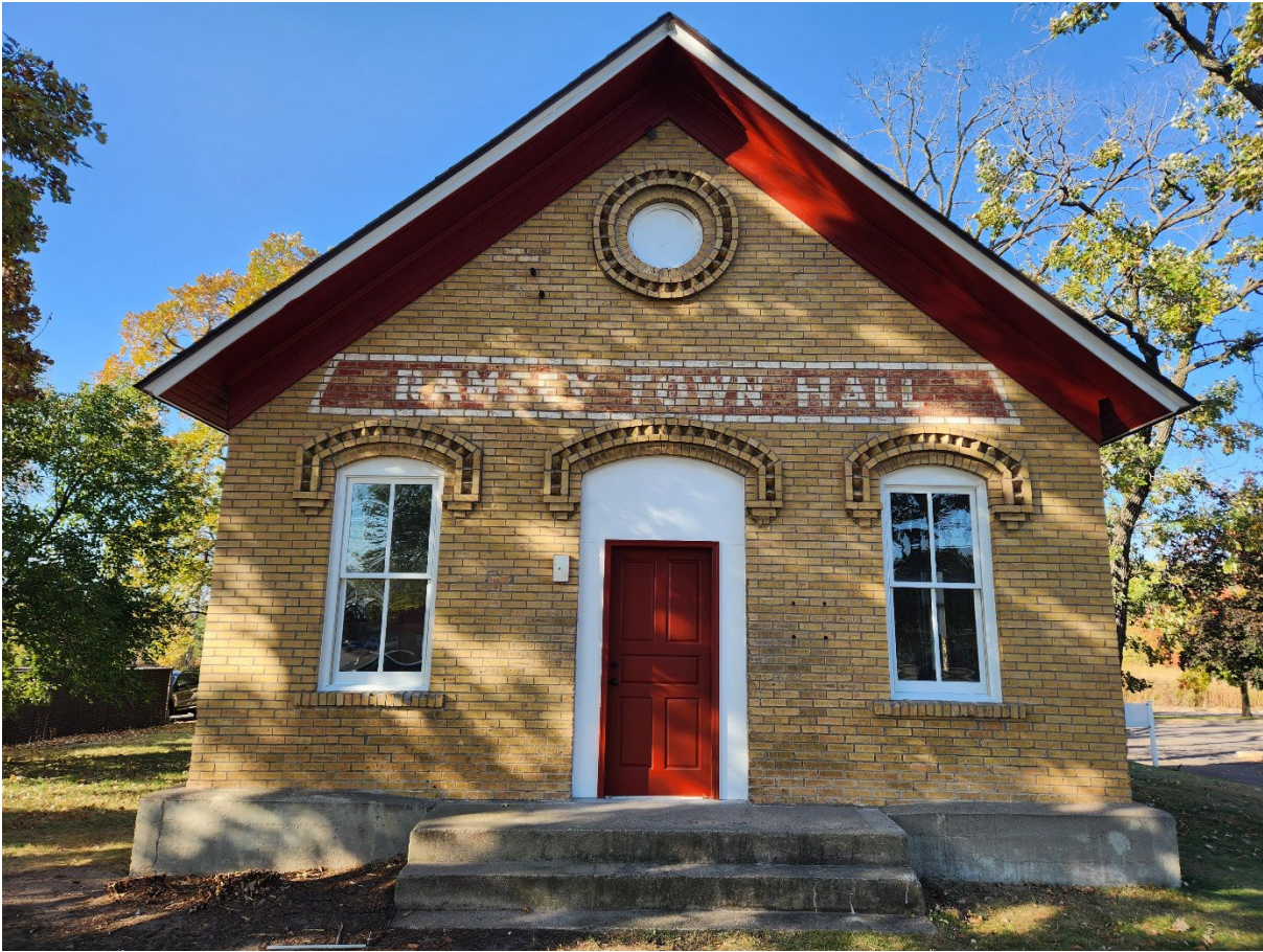
Window Fixed / Windows Painted / Soffits (repaired)
