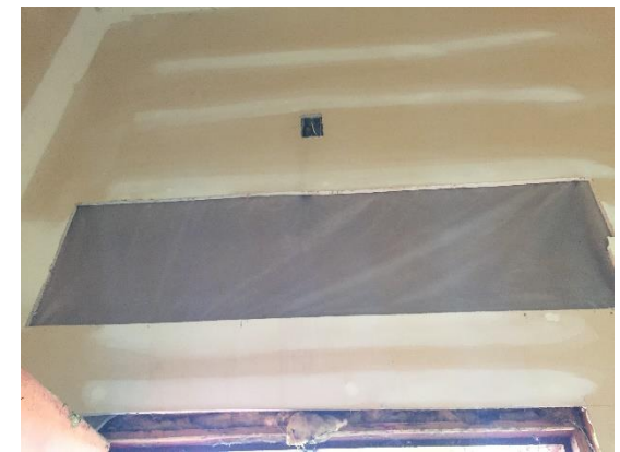
Figure 32 – Opening Above Entry
