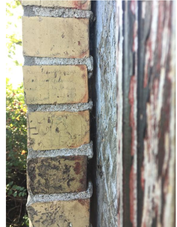
Figure 10 – Accessible Gap Behind Brick
