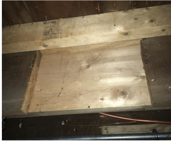
Figure 44 – Replacement Floor Joist
