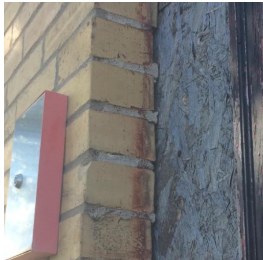
Figure 7 – Red Paint on Side Framing
