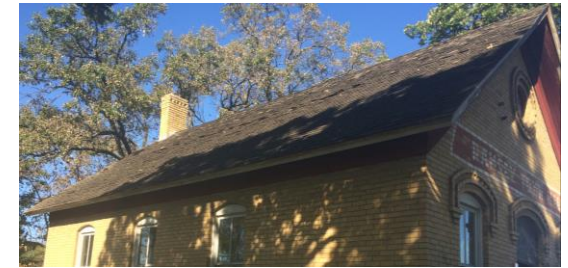
Figure 28 – Asphalt Shingles
