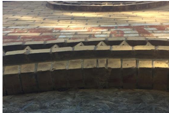
Figure 6 – Red Paint on Overhead Framing
