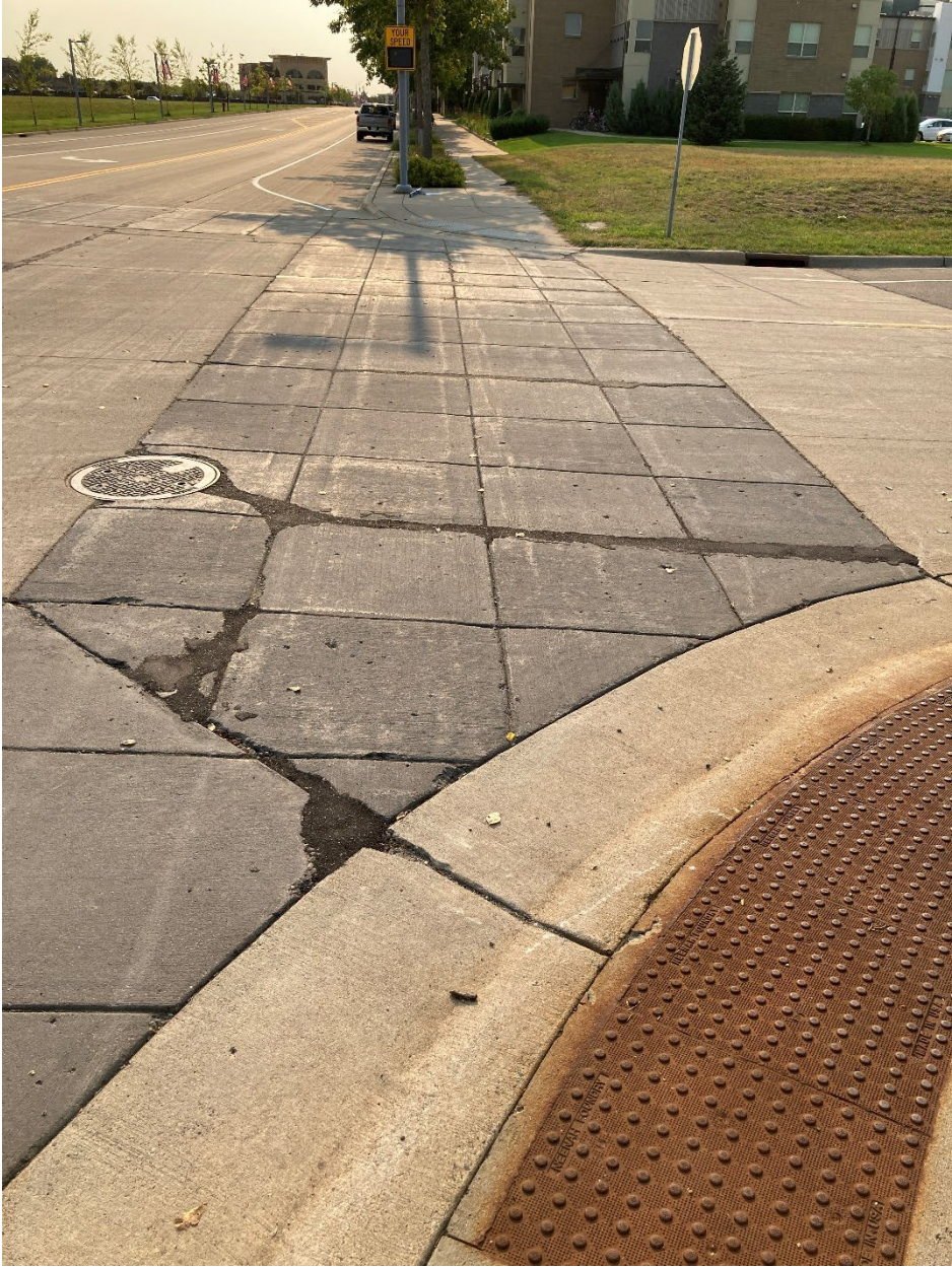
SW Quad Sunwood Drive & Yolite Street; Facing East
