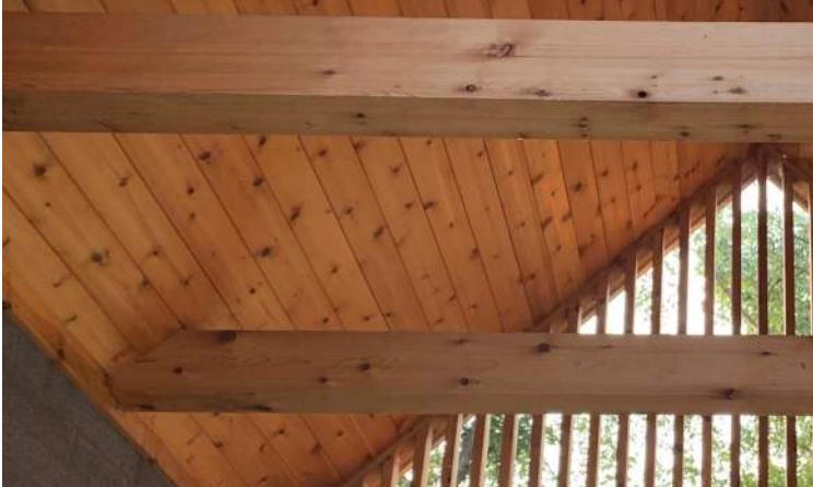
T&G Cedar Roof Underside Decking
