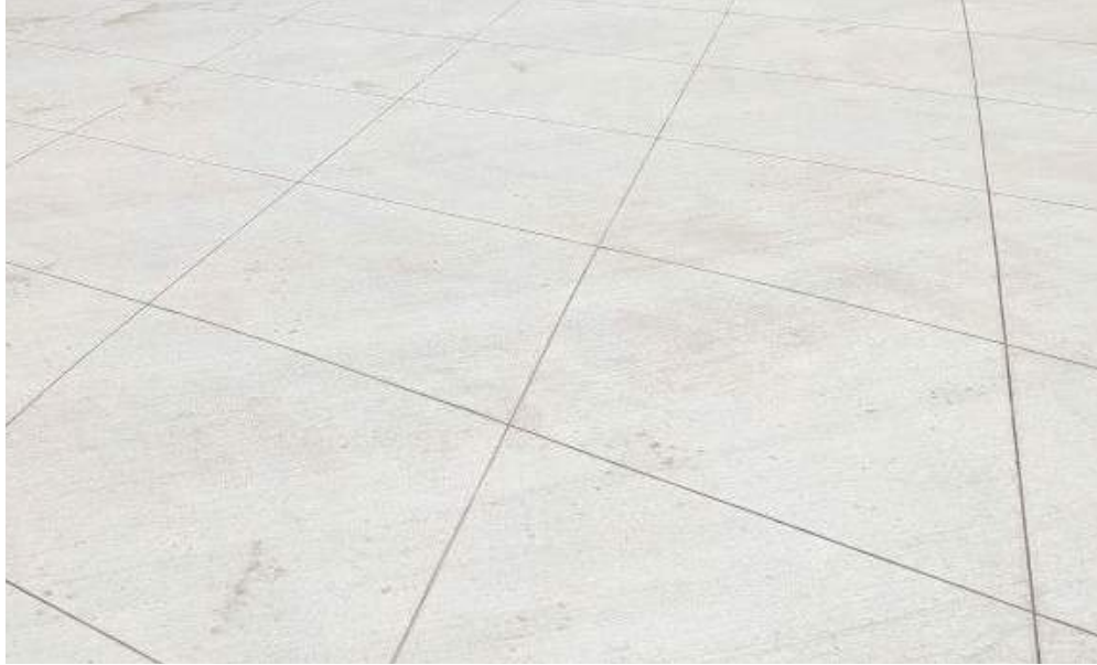
Concrete Paving - Standard Gray Broomed
