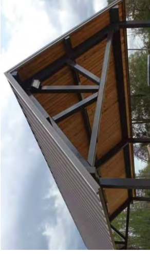
Standing Seam Metal Roof
