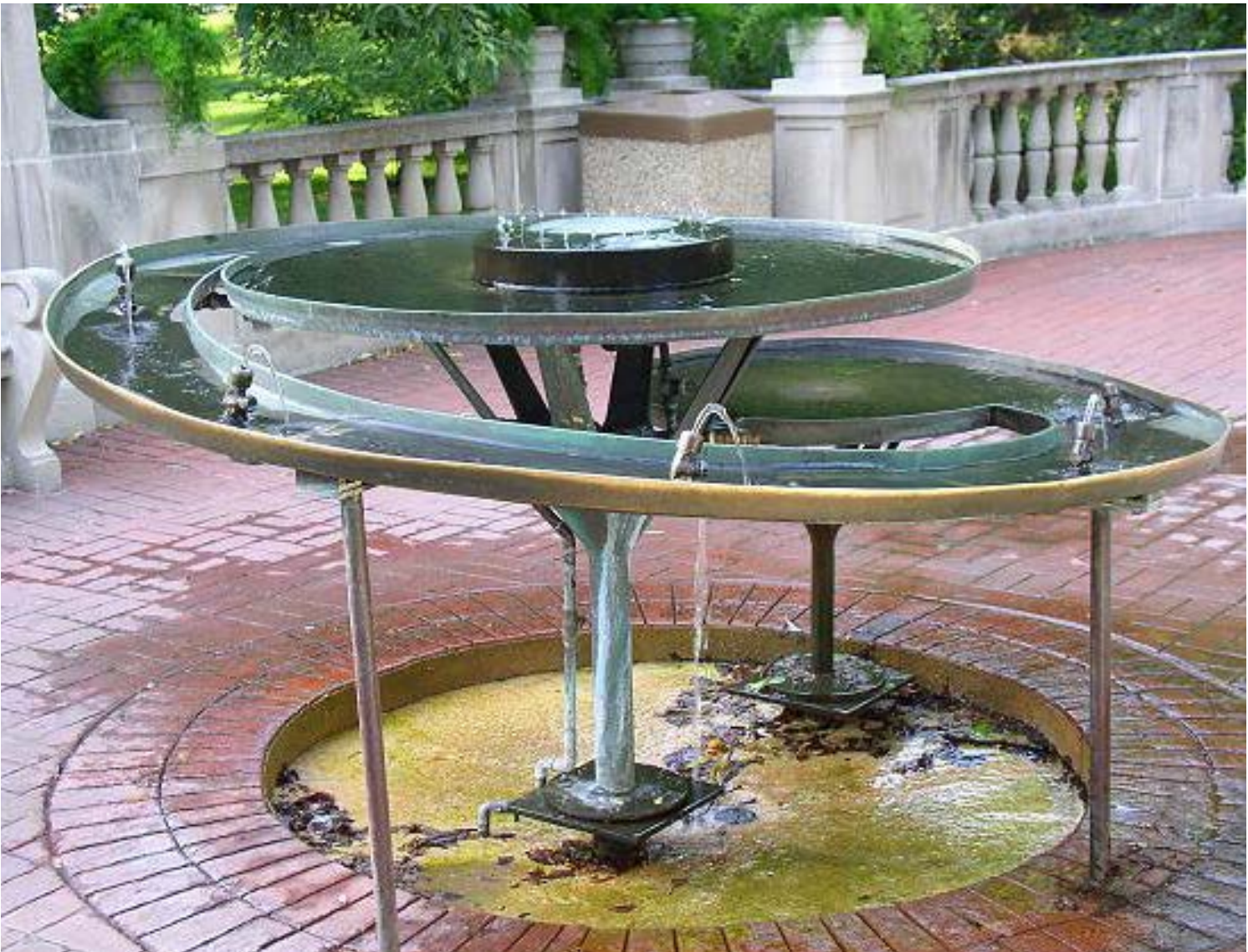
Designed in 1962 by architect Gyo Obata, this sculptural copper fountain once stood outside the Discovery Corner Railroad station at the Saint Louis Zoo. Photo by Flickr user Jer
