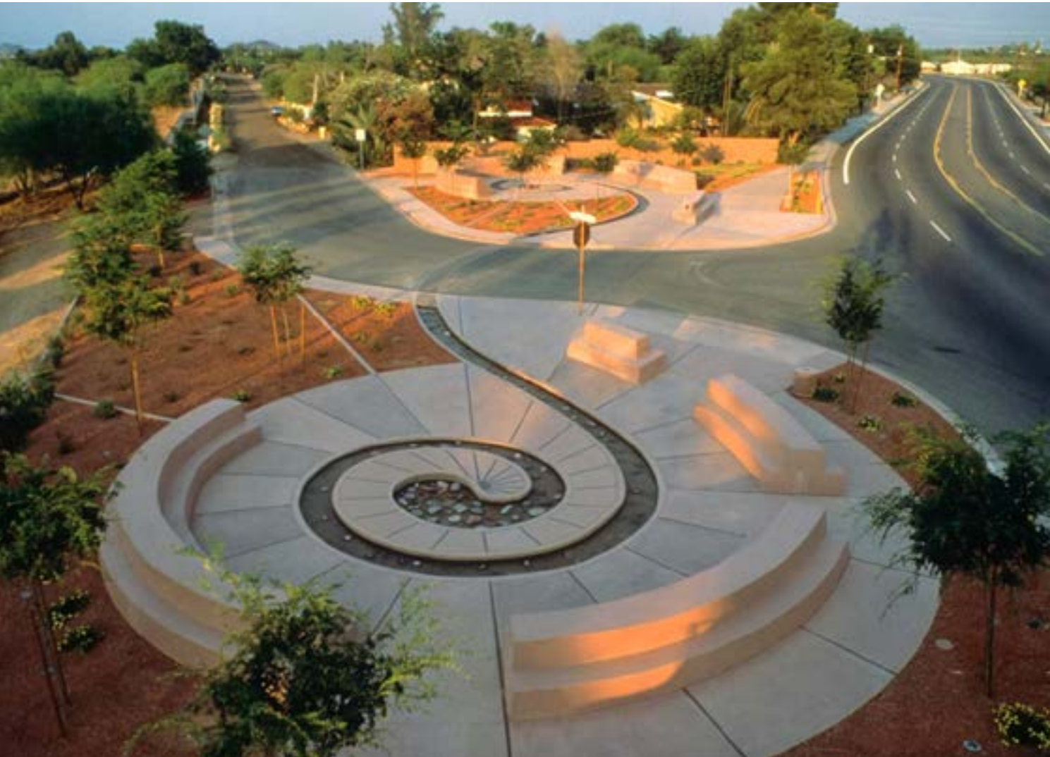
The Spiral channel in the piece draws water from the road and returns it to a local canal. Photo by Greg Smith.
