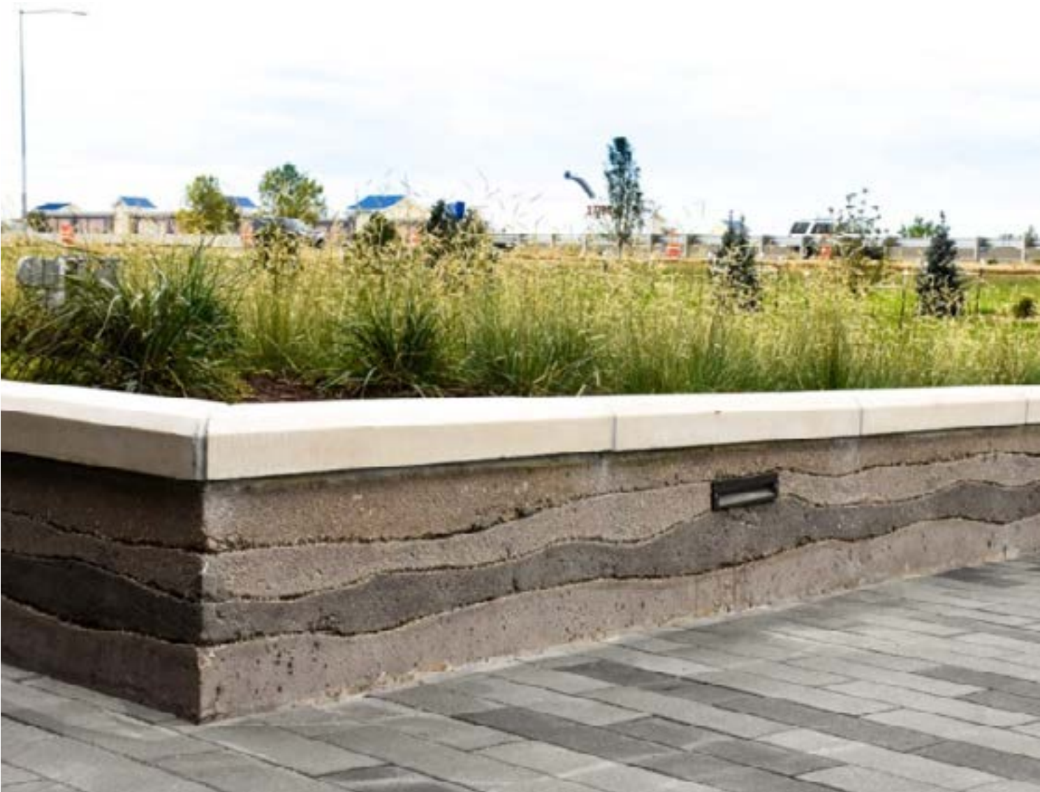
Sedimentary walls compress layers of concrete to mimic the passage of millennia, capturing the look of rammed earth in a permanent form.
