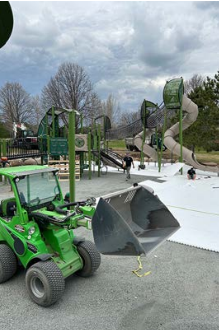
Construction of the new Central Park Playground, May 2025. While core funding supported the playground build, musical play elements were incorporated into the design, adding a subtle layer of community art that blends creativity, sound, and play.
