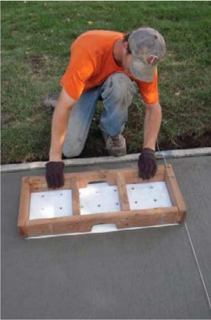
Each year, new poems are stamped during sidewalk repairs, making literature a routine part of city maintenance. Photo sourced from Public Art St. Paul
