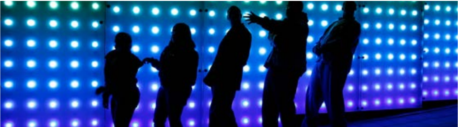
LED panels conceal utility equipment while transforming Raleigh’s City Plaza into a colorful, shifting light environment. Photos courtesy of Susan Harbage Page
