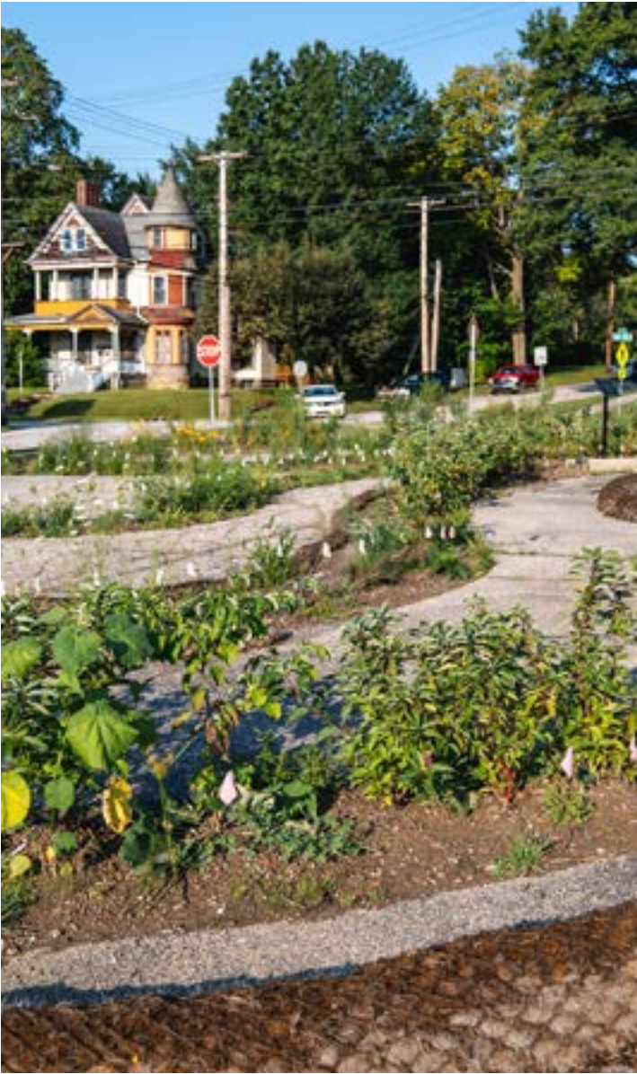
This project includes 515 feet of swales, 30" wide and 24" deep, in the southwest corner of the parking lot.
