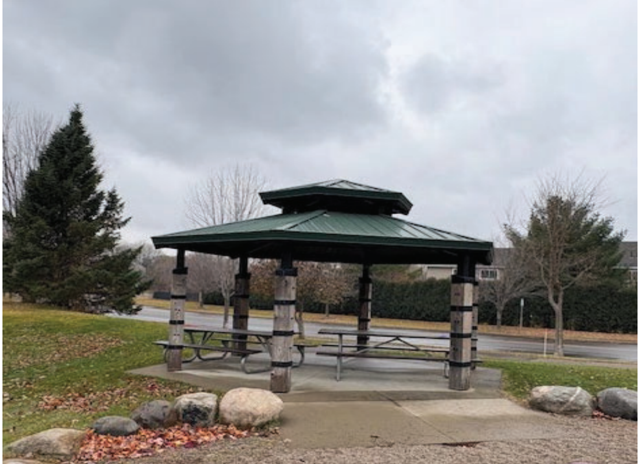
Pavilion and concrete to be protected.
