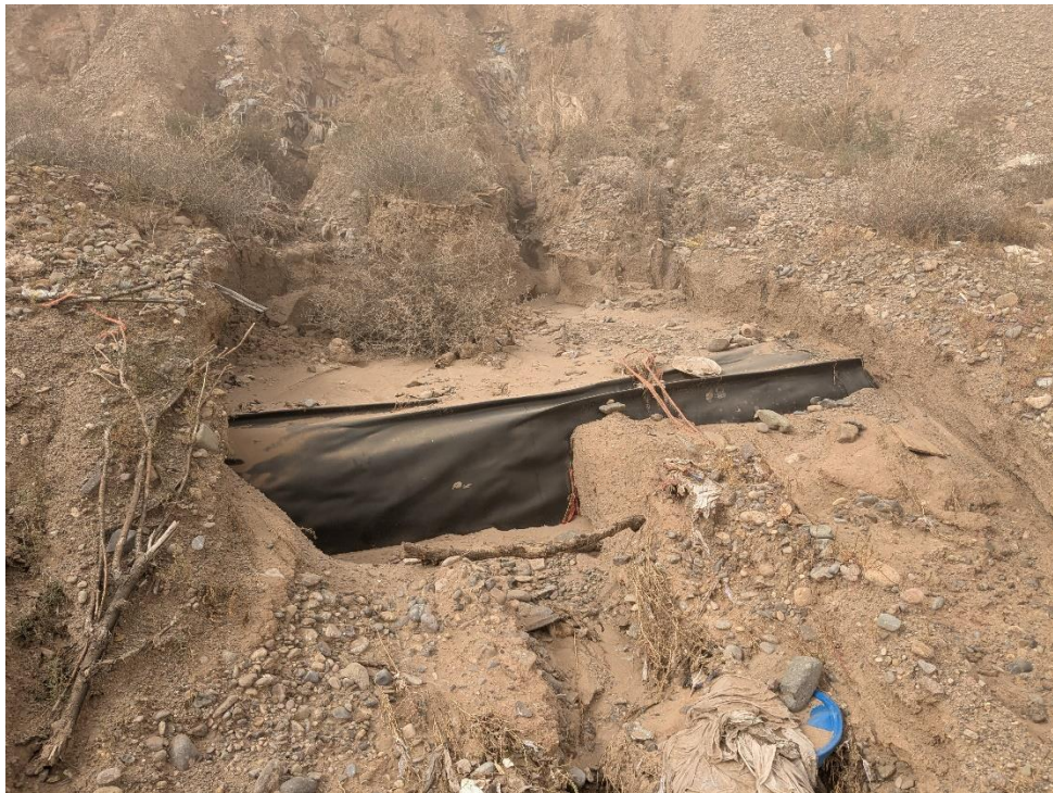
Photo 11. Anchor Trench of Unit 5A liner exposed on Unit 4 eastern-facing side slope
