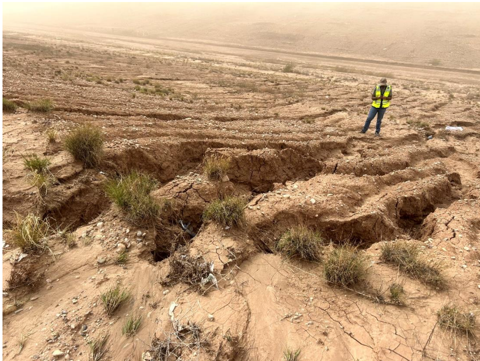
Photo 7. Erosional channels on western-facing side slope of Unit 3 side slope
