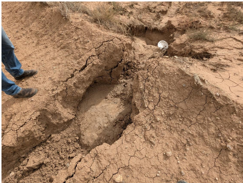
Photo 8. Exposed compacted clay layer, Unit 3 side slope
