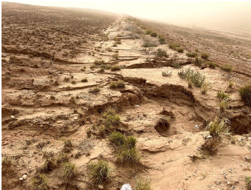
Photo 9. Damage to existing graded stormwater flow path atop Unit 3.
