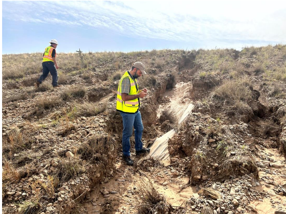
Photo 1. Geotextile exposed along northern side slope of Unit 1 Cell
