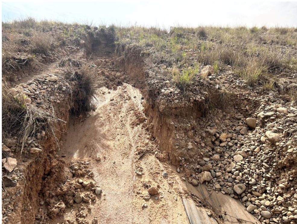
Photo 2. Geotextile underlying vegetative top cover on northern Unit 1 slope
