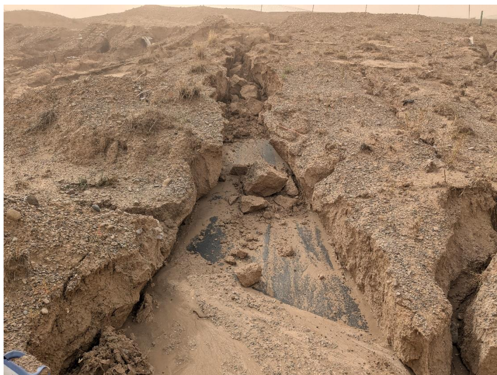
Photo 12. Exposed Unit 5A liner southwest of tie-in with Unit 4
