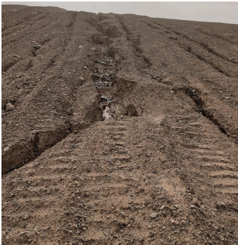
Photo 10. Channel and erosion of buried waste material on the northern face of Unit 4.
