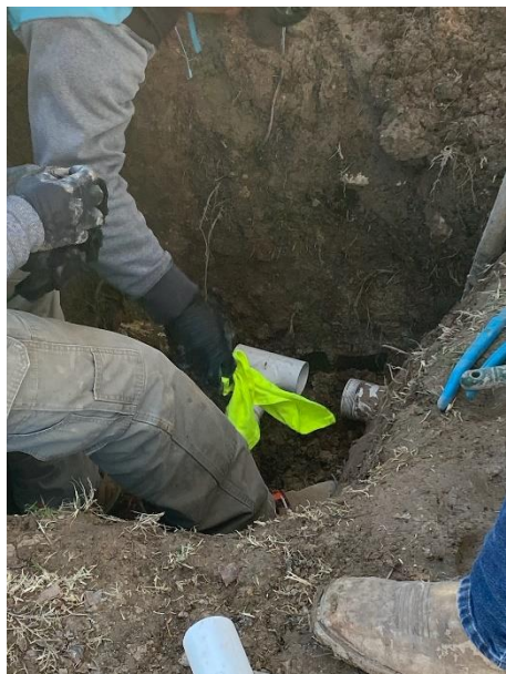
Left: Water line break in the longhorn enclosure. Dug up and repaired by the zoo grounds team and the parks department irrigation team.
