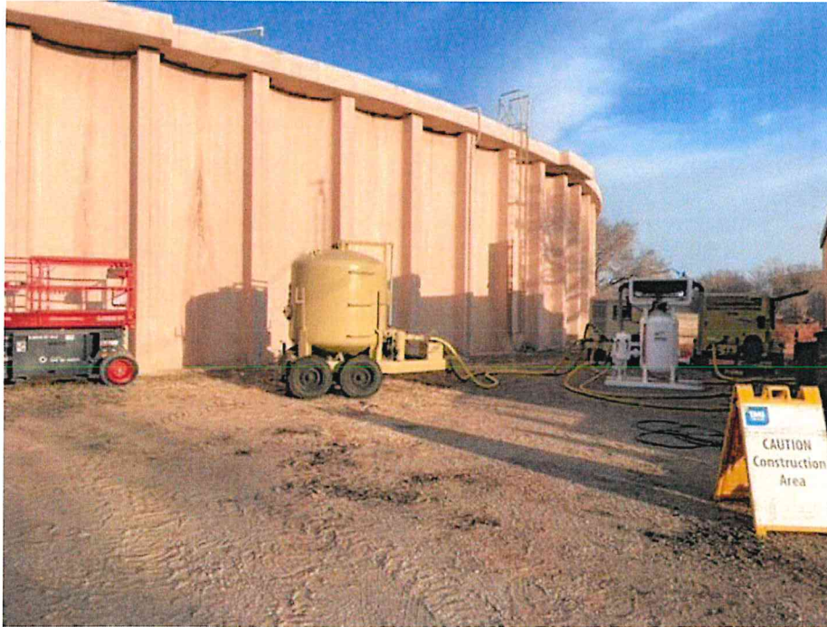
7,500,000 Gallon Concrete Ground Storage Tank "South Country Club Tank" City of Roswell Roswell, New Mexico
