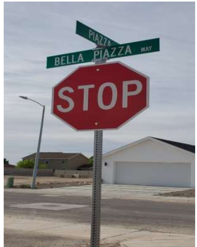
Installing new street and stop sign
