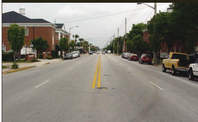
Figure 1. Photo. Four-lane configuration before road diet.
