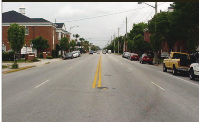
Figure 1. Photo. Four-lane configuration before road diet.
