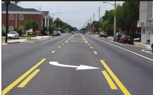
Figure 2. Photo. Three-lane configuration after road diet.
